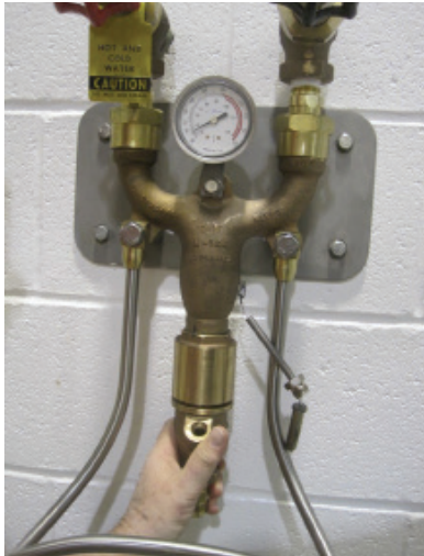
4. Remove Lower Thermostat Housing
