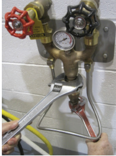
2. Loosen Lower Thermostat Housing
