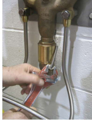
3. Remove Thermostat bulb
