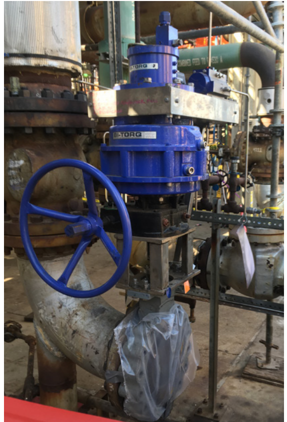
R-EBV ABOUT TO BE INSTALLED ON A HYDROSPHERE
